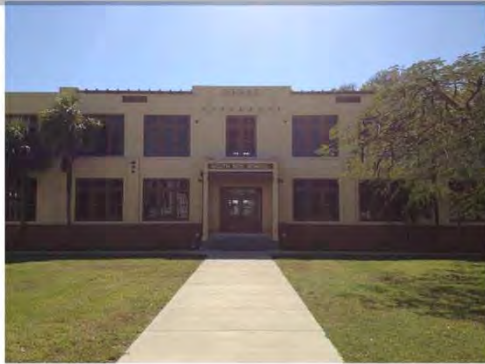
N.E. FACADE OF SCHOOL
