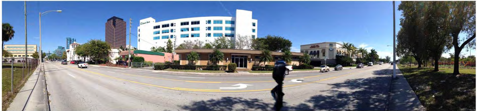
PANORAMIC VIEW FROM ANDREWS AVENUE LOOKING EAST
