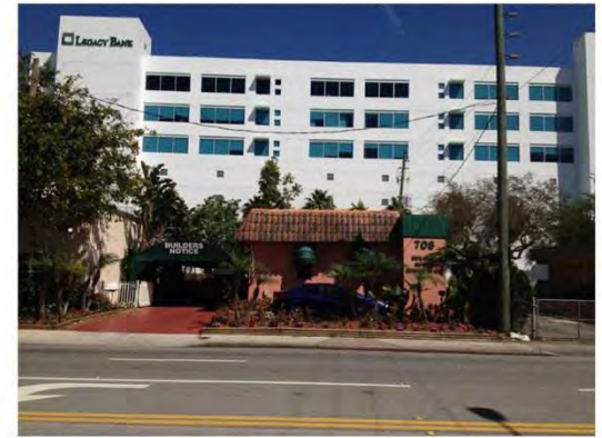
STRUCTURE EAST OF PUBLIC PARK
