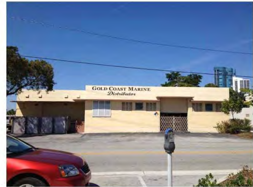
STRUCTURE NORTH OF PUMP HOUSE
