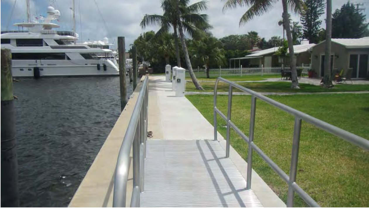
1. North corner of the subject site, facing south. Note existing seawall.
