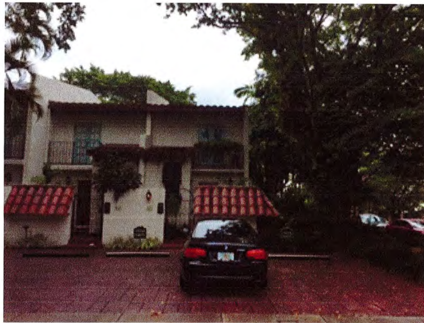
VIEW FROM CANAL TO 827
