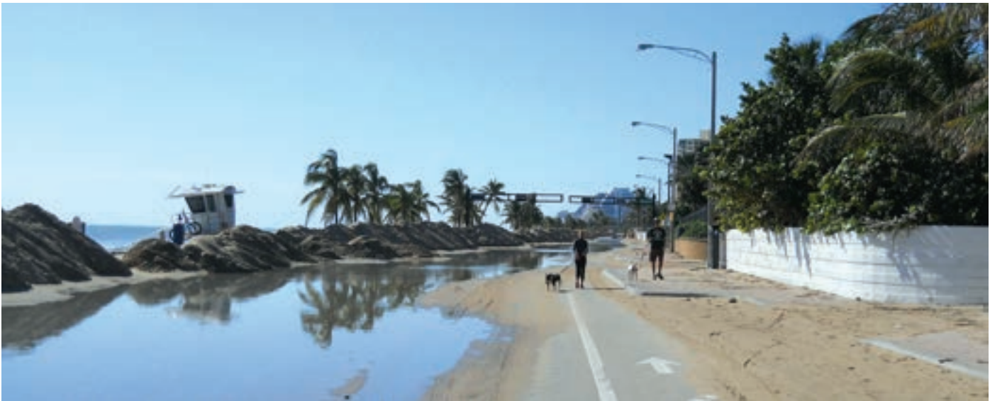
State Road A1A after Hurricane Sandy
