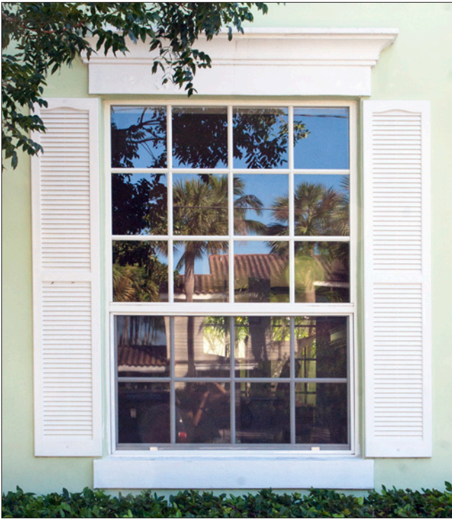
Shutters should be operable and proportioned to fit the window. The shutters in this example are fastened to the face of the building and too narrow for the window opening.
