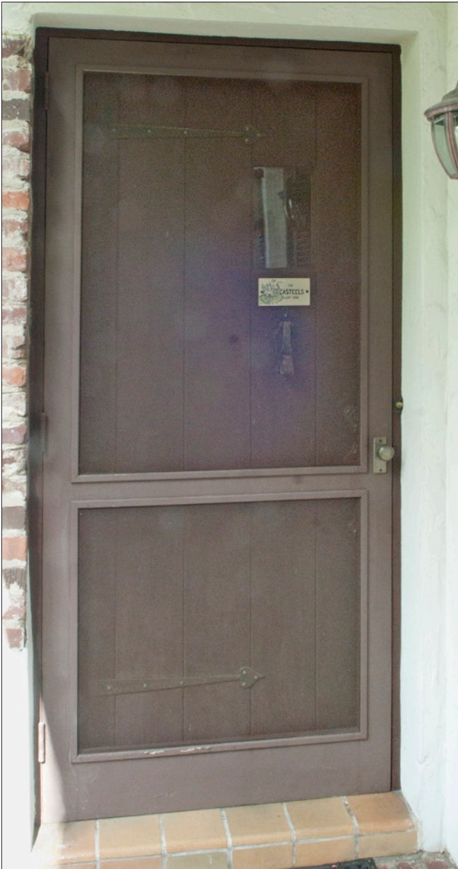
This screen door includes large screened areas that allow the historic entrance door beyond to remain visible. The screen door is also painted to match the color of the wood door and surrounding trim.
