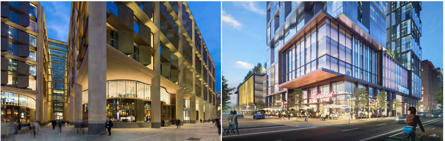
High quality building design, illumination features, and parking garage screening. Sources: awards.lighting.co.uk/winners-2018/ & www.pittsburghmagazine.com/downtown-plans-from-parking-garage-to-luxury-condos/ (rendering courtesy AE7 Pittsburgh LLC, 2017)
