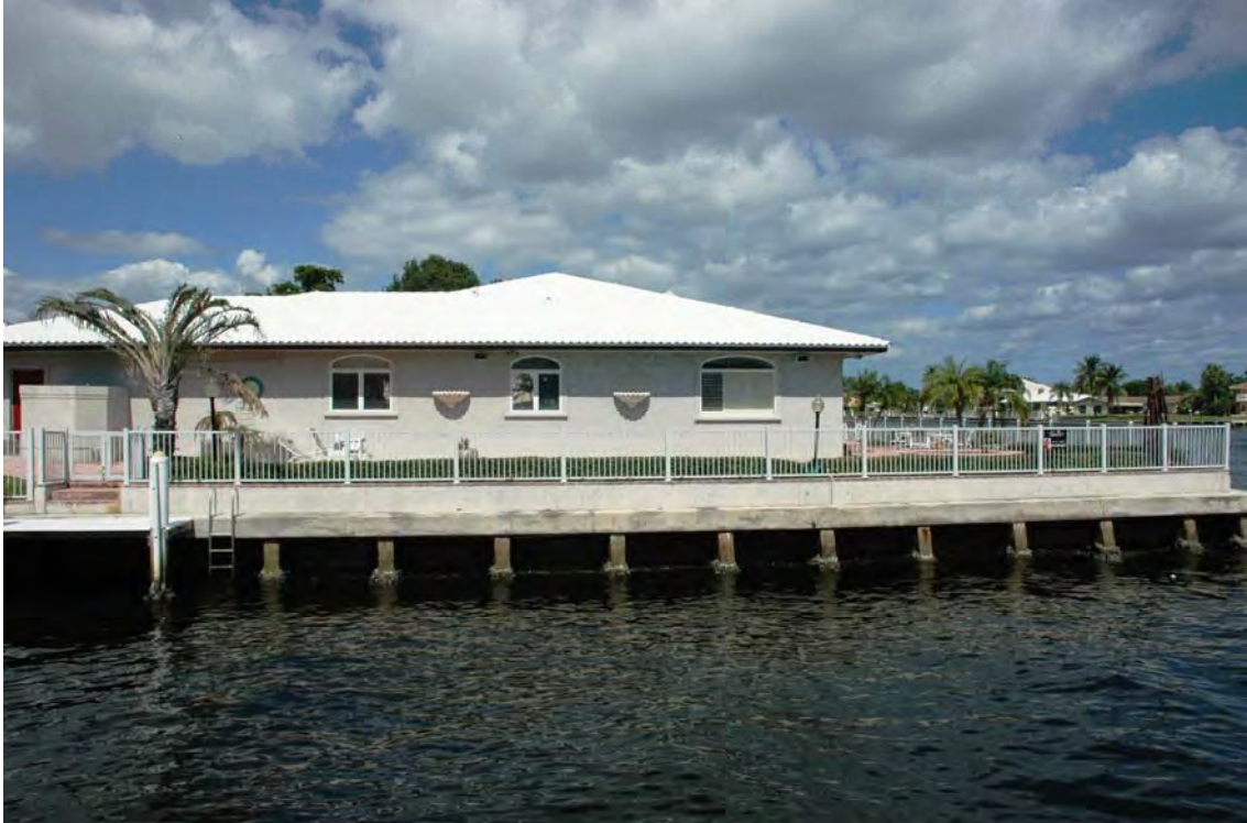
3. Western property boundary, facing north along the canal.
