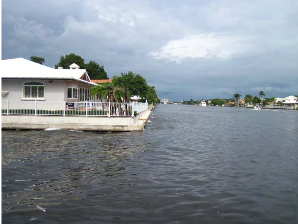
5. Eastern property boundary, facing north along the ICWW.
