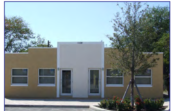
1108 Sistrunk Boulevard, After
