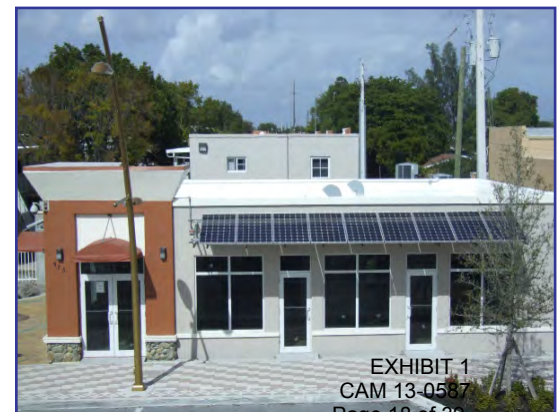
915 Sistrunk Boulevard, After
