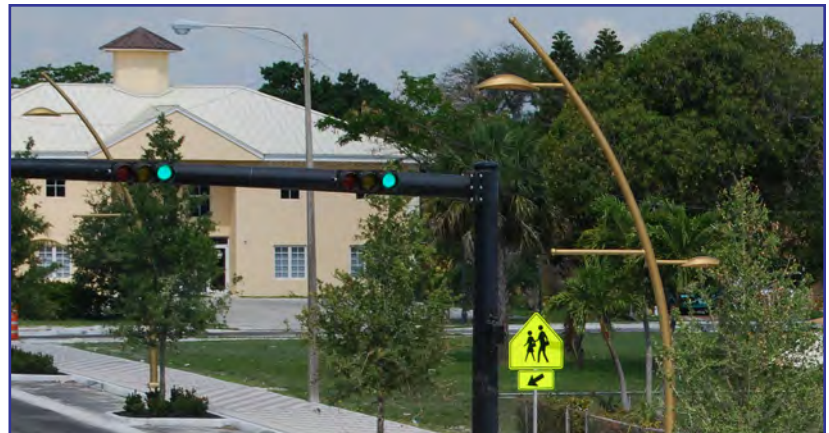
Sistrunk Boulevard Infrastructure Project
