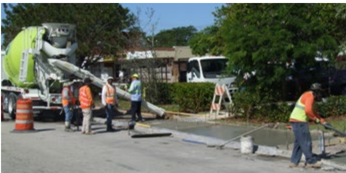
NE 13 Street Improvements
