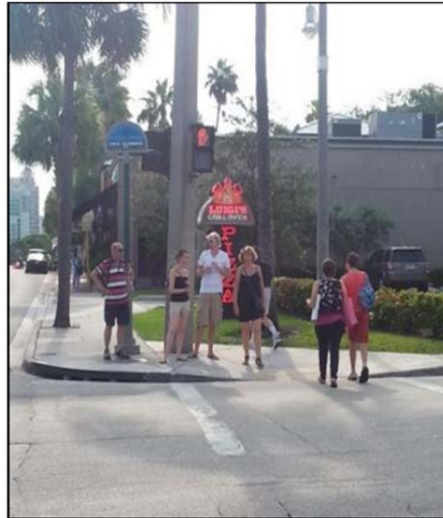
Worn crosswalk markings across 15 th Ave.
