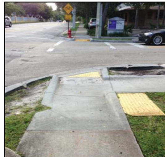
Single-unit truck turning wide at Broward Blvd; damage to curb and sidewalk
