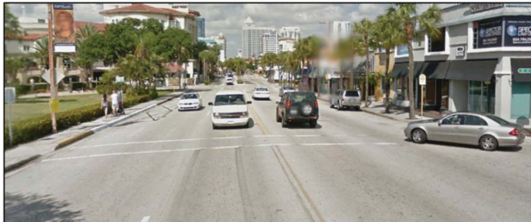
Worn mid-block crosswalk markings – opportunity to provide enhanced crosswalk
