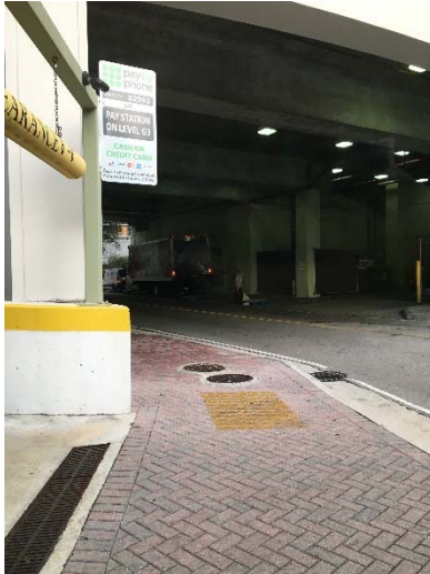
Loading zone under Riverside Hotel parking garage.
