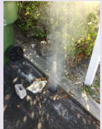
Missing/damaged clean-out caps
