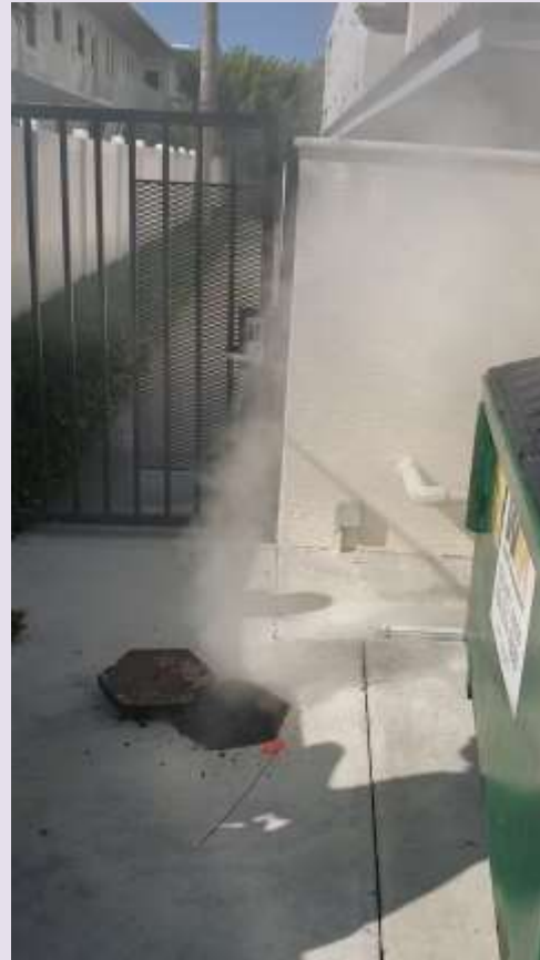
Missing/damaged clean-out caps
