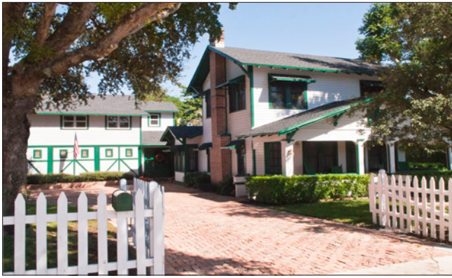
Historic secondary buildings should be maintained. This example has similar design elements and materials as the main house.
