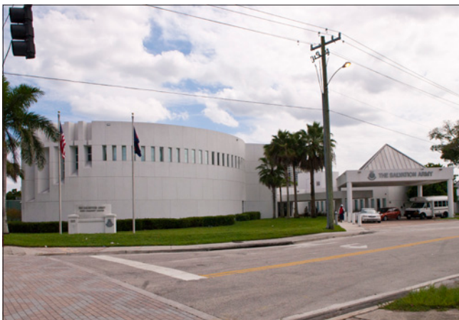
The new building is located at the corner of a major intersection with the drop-off area located on a secondary street and parking to the rear. The mass of the building is broken down into several volumes, reducing its perceived size.
