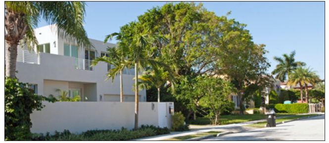
The modern house has a similar scale and setback as its neighbors.
