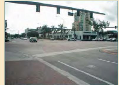
[Figure 4.36] A large curb radius causes longer, less safe pedestrian crossing distances
