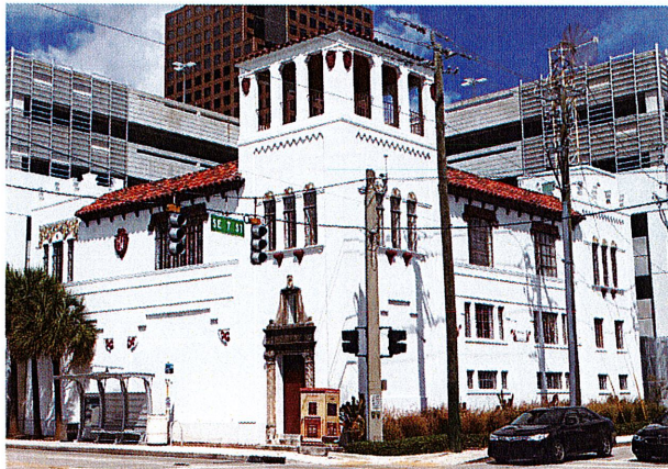
Photo of Existing Conditions
