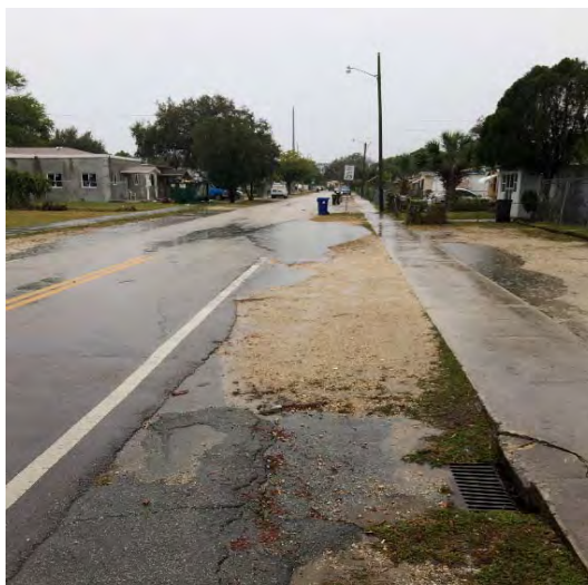
NW 15th Way between NW 5th Street and NW 6th Street on February 22, 2017. Example of poorly graded/paved swales.
