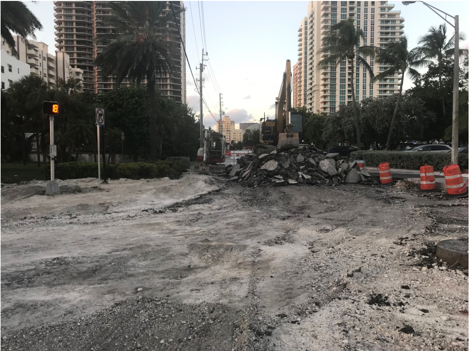
FESTIVAL STREET PROGRESS PHOTO TAKEN ON 10-14-2019 (SEABREEZE AND LAS OLAS INTERSECTION)
