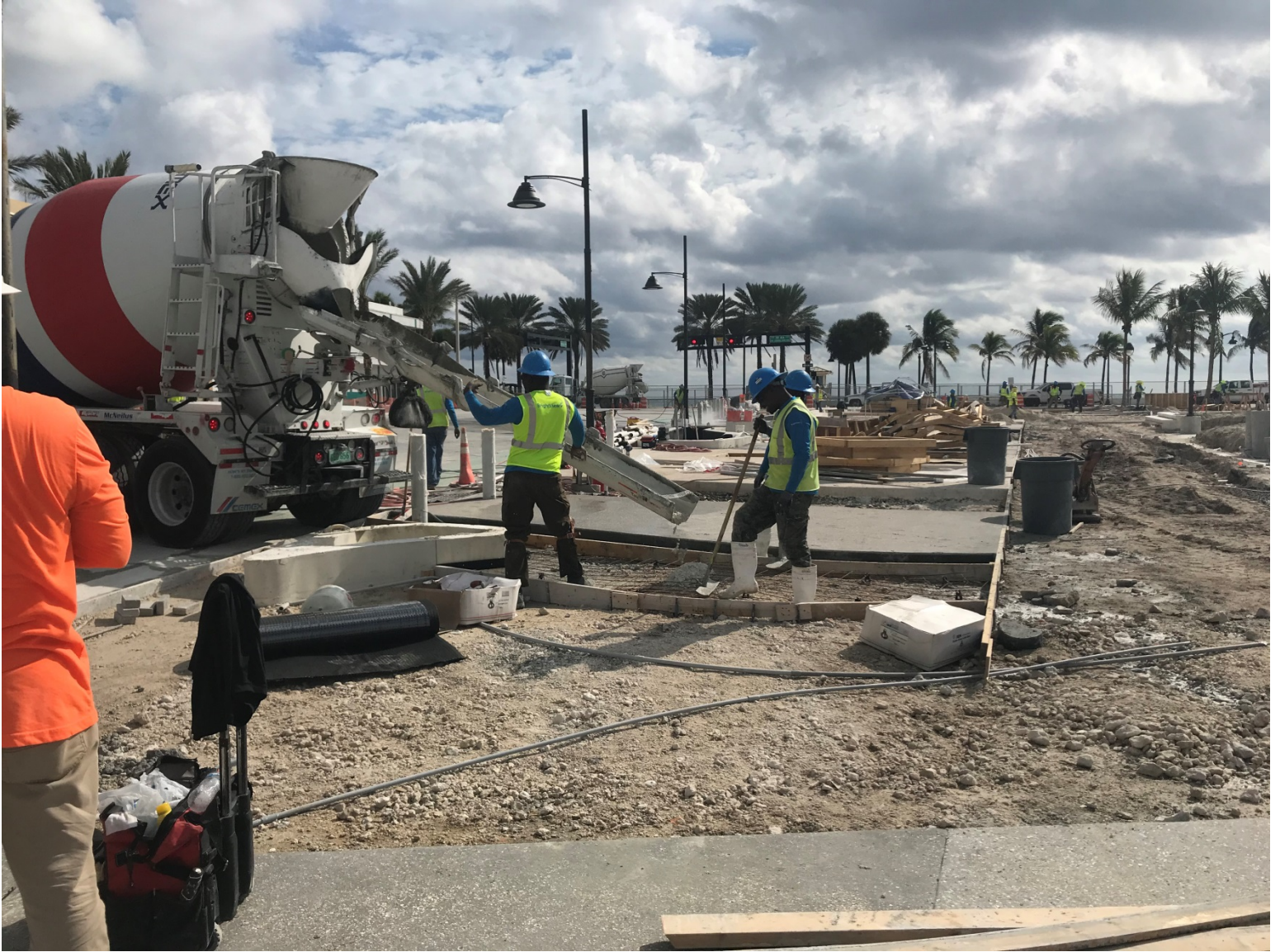
OCEANSIDE PARK PROGRESS PHOTO 10-15-2019 (SIDEWALK POUR FACING EAST)
