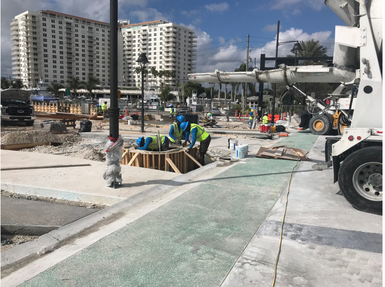
OCEANSIDE PARK PROGRESS PHOTO 10-15-2019 (STEM WALL POUR FACING WEST)
