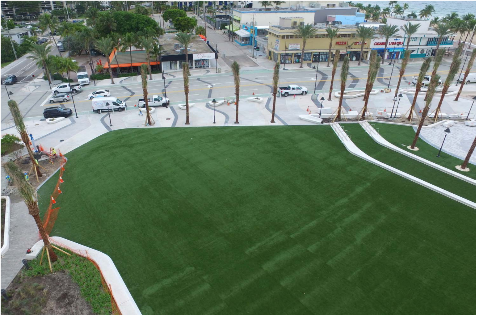
LAS OLAS PROJECT AERIAL PHOTO TAKEN ON 11-21-2019
