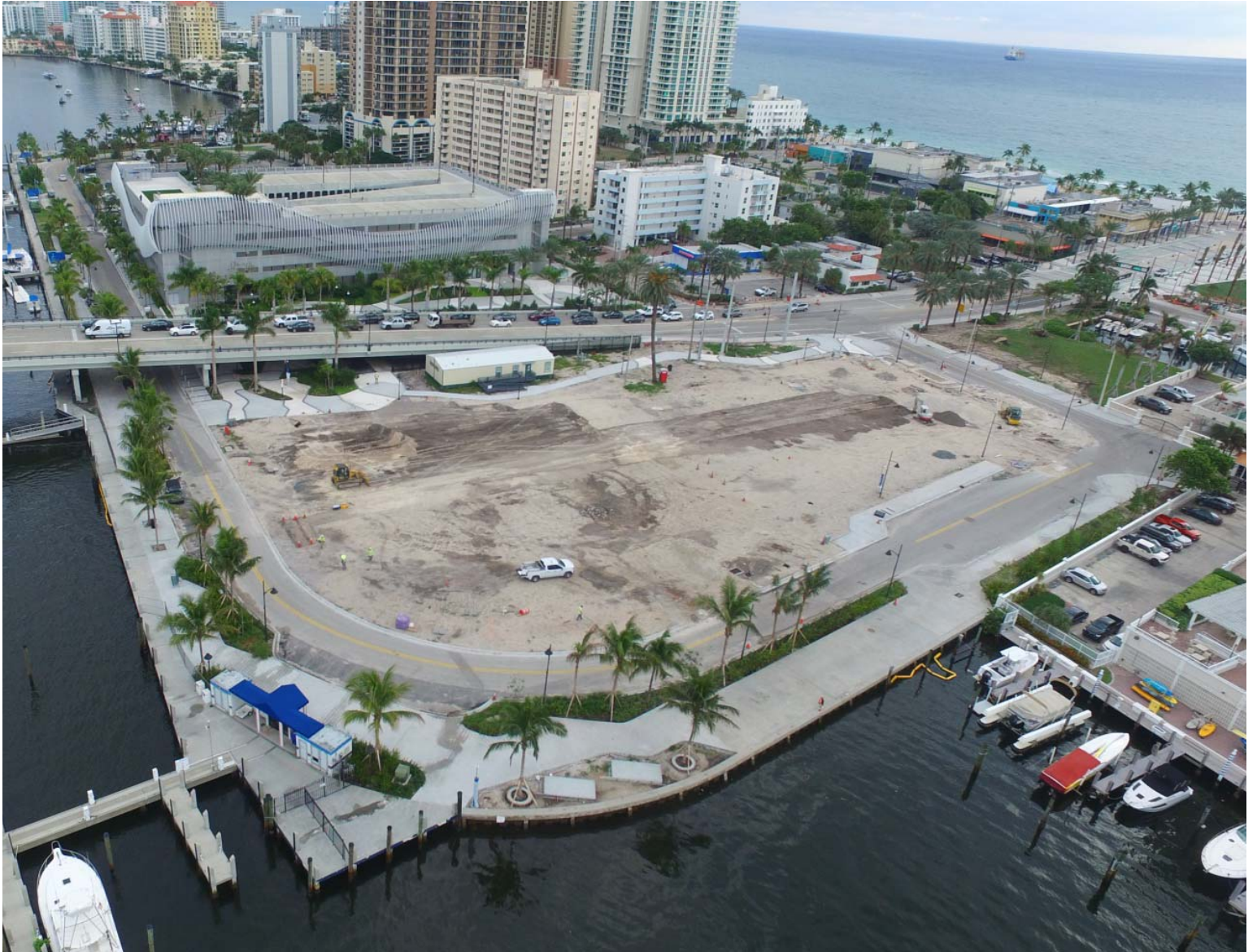
LAS OLAS PROJECT AERIAL PHOTO TAKEN ON 11-21-2019
