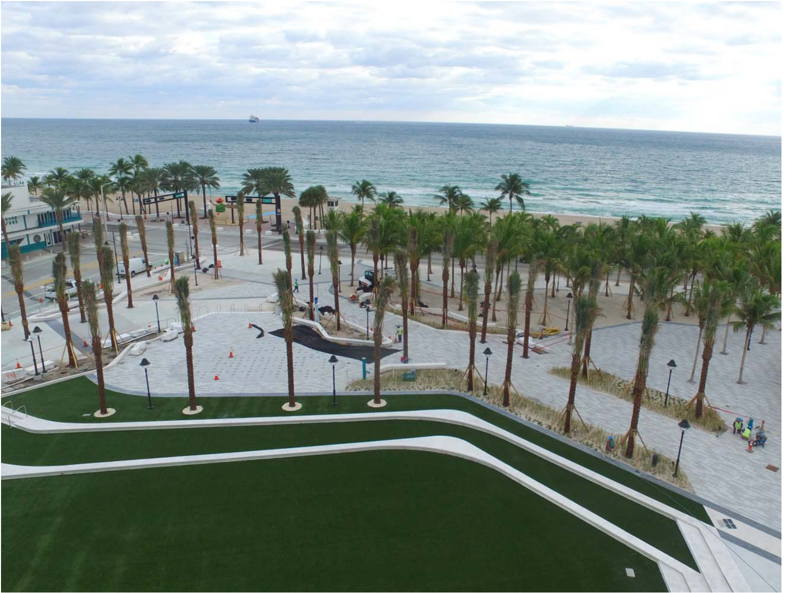
LAS OLAS PROJECT AERIAL PHOTO TAKEN ON 11-21-2019
