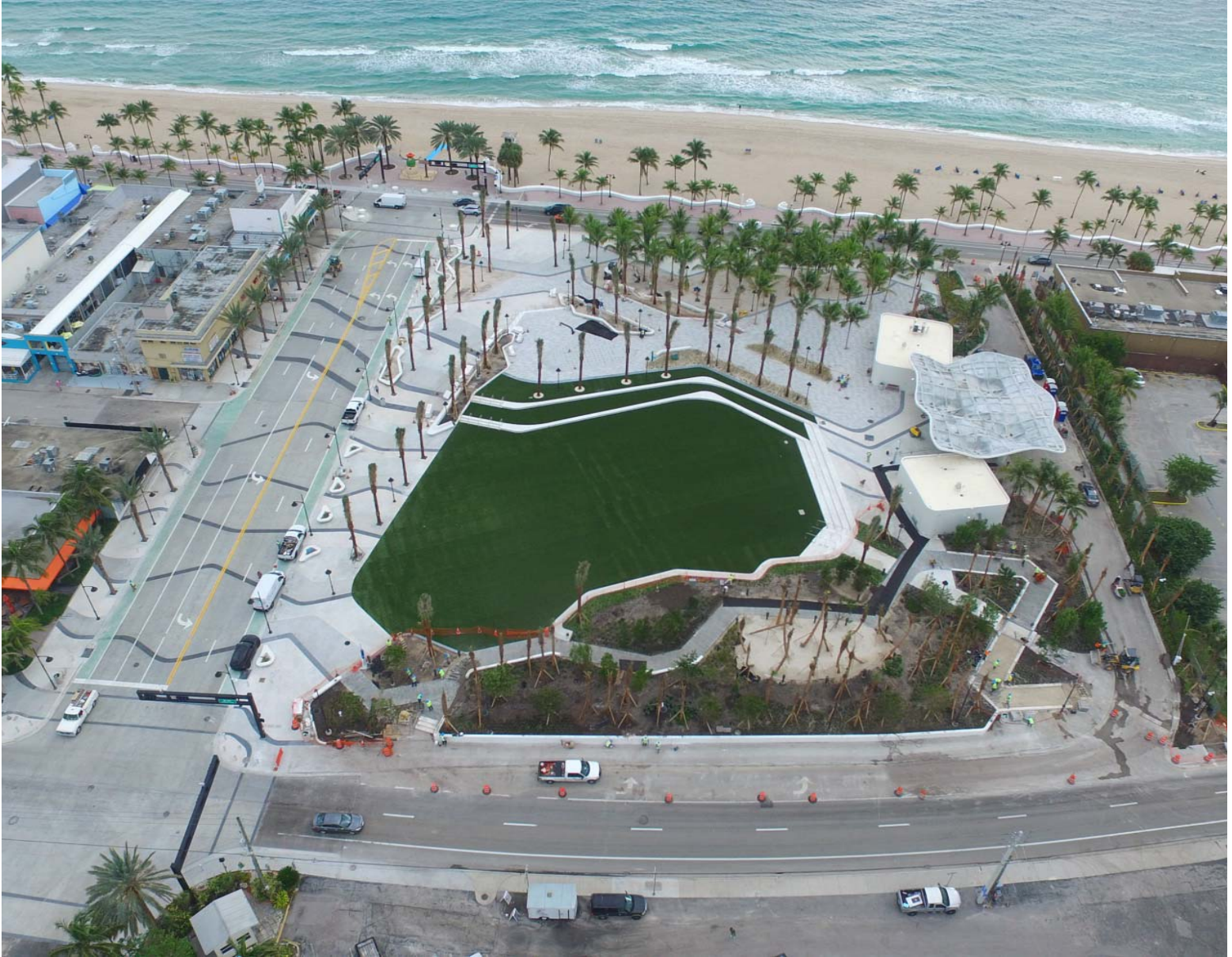
LAS OLAS PROJECT AERIAL PHOTO TAKEN ON 11-21-2019
