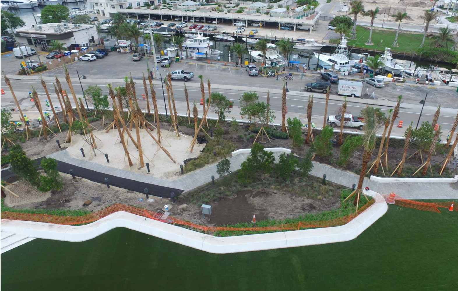
LAS OLAS PROJECT AERIAL PHOTO TAKEN ON 11-21-2019
