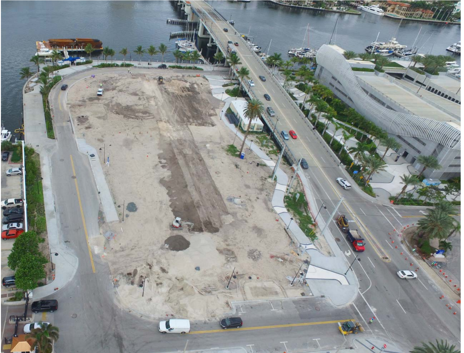
LAS OLAS PROJECT AERIAL PHOTO TAKEN ON 11-21-2019
