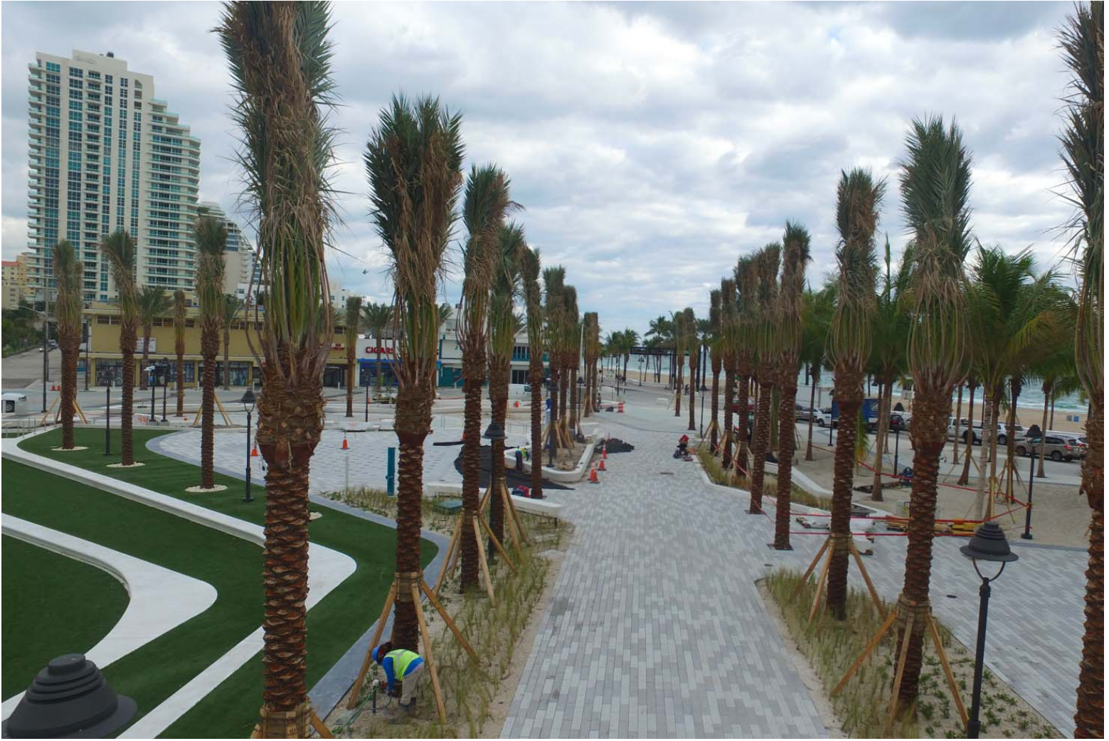
LAS OLAS PROJECT AERIAL PHOTO TAKEN ON 11-21-2019
