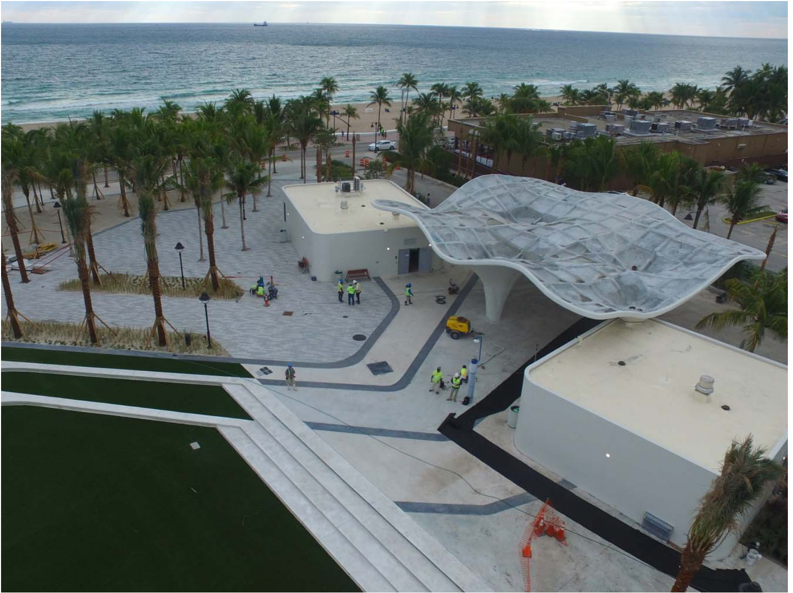
LAS OLAS PROJECT AERIAL PHOTO TAKEN ON 11-21-2019
