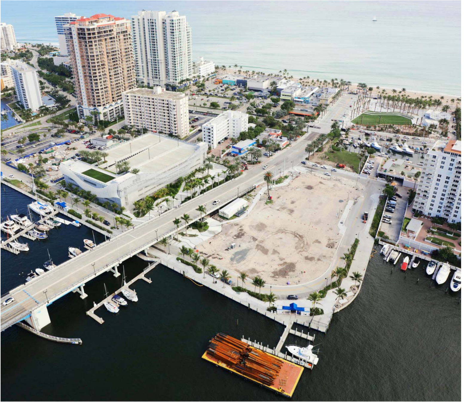
LAS OLAS PROJECT AERIAL PHOTO TAKEN ON 11-19-2019
