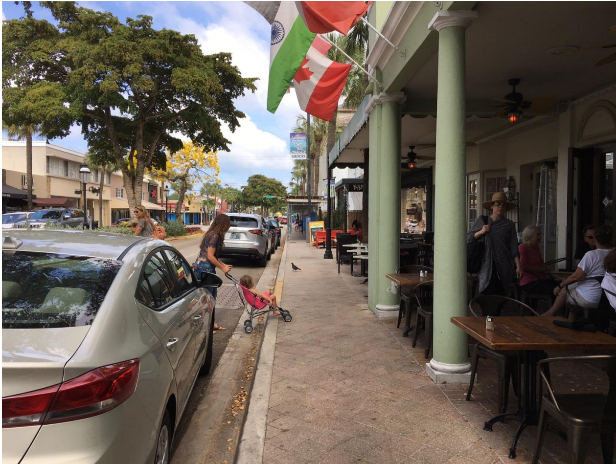
Lack of ADA ramps creates issues using midblock crossings
