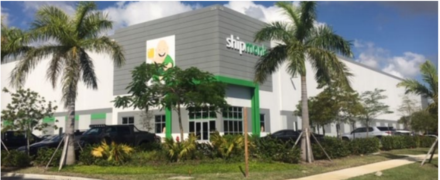
Shipmonk Completed Project - 201 NW 22 Avenue
