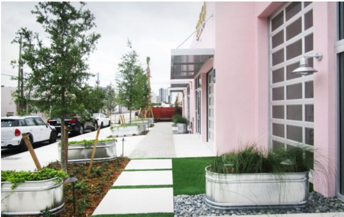
Completion of 835 and 837 NE 2 Avenue Exterior
