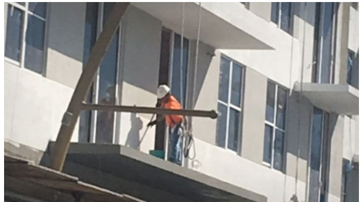
Six13 Project Under Construction
