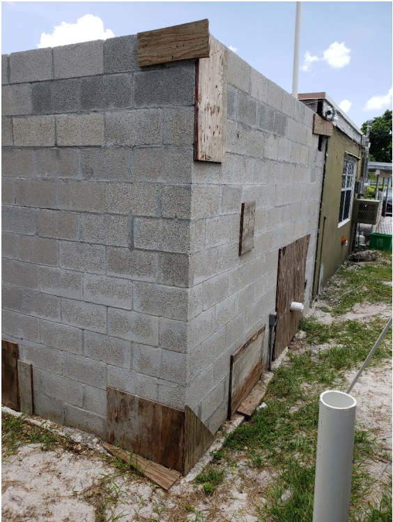
Rear Addition – East Elevation
