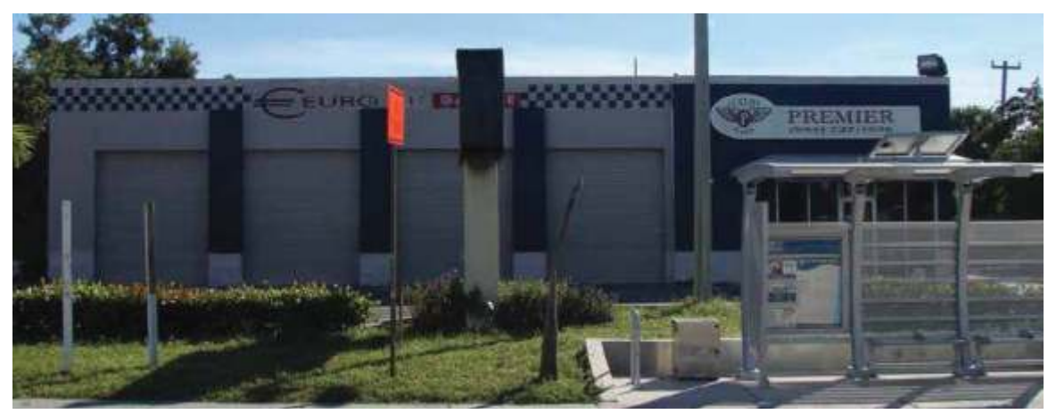
Reference: Existing Condition
