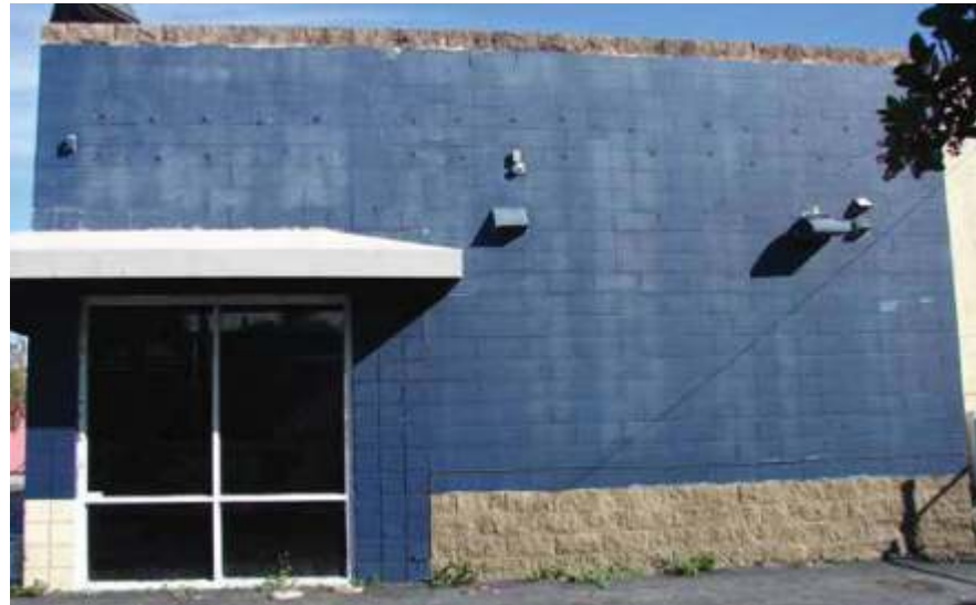
Reference: Existing Condition
