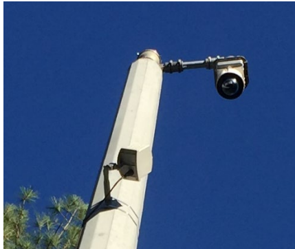
ROADWAY CCTV CAMERA AND TRAFFIC SENSOR (MDVS)
