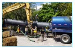
on the northern end of the project, Murphy Pipeline has completed fusing 1,100 feet of pipe that will be installed on NE 18 Street between NE 15 and NE 17 Terrace, and is mobilizing to begin drilling a pilot hole that will serve as the initial underground pathway for the pipe. In addition, crews are continuing to drill an underground pathway along Bayview Drive from NE 30 Street to NE 37 Street in preparation for the installation of 2,600 feet of pipe.
