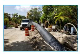
Two contractors are working on the project simultaneously to fast-track construction. Murphy Pipeline is installing the northern portion of the pipe and David Mancini & Sons, Inc. is installing the southern portion. Both companies are using directional boring, which expedites installation by eliminating the need to dig up entire streets, minimizes disruption to the neighborhoods and traffic flow, and decreases the amount of time needed for restoration work.
