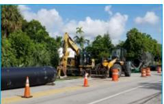
According to Mancini, the half-mile segment of 54-inch high density polyethylene (HDPE) pipe set a world record for the longest and largest directionally drilled pressurized sewer pipe installation, surpassing the company's previous record of 3,000 feet that was set in Miami Beach. The Fort Lauderdale operation required more than 23 sections of pipe to be fused together as it was being pulled underground.
