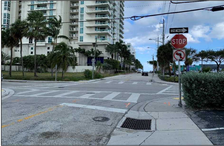
Photograph 4: Eastbound Poinsettia Street approaching Seabreeze Boulevard
