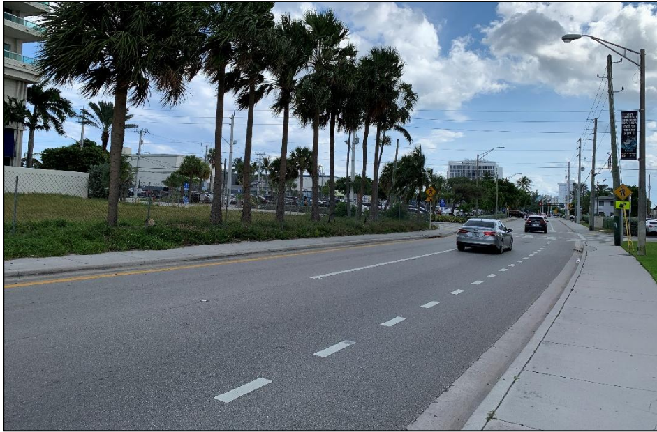
Photograph 2: Southbound Seabreeze Boulevard approaching Poinsettia Street
