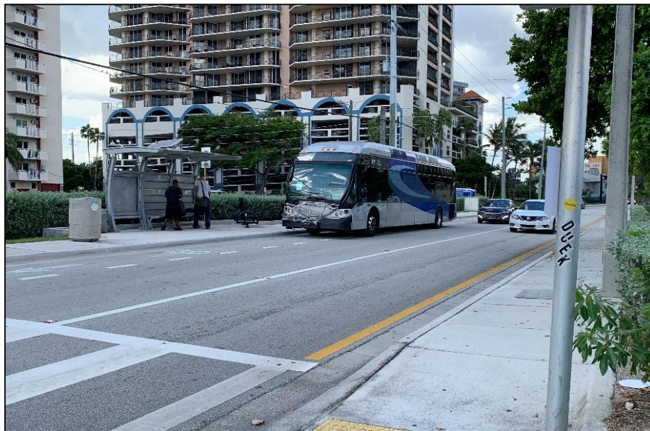
Photograph 9: Bus Stop along Seabreeze Boulevard South of Poinsettia Street (looking north)
