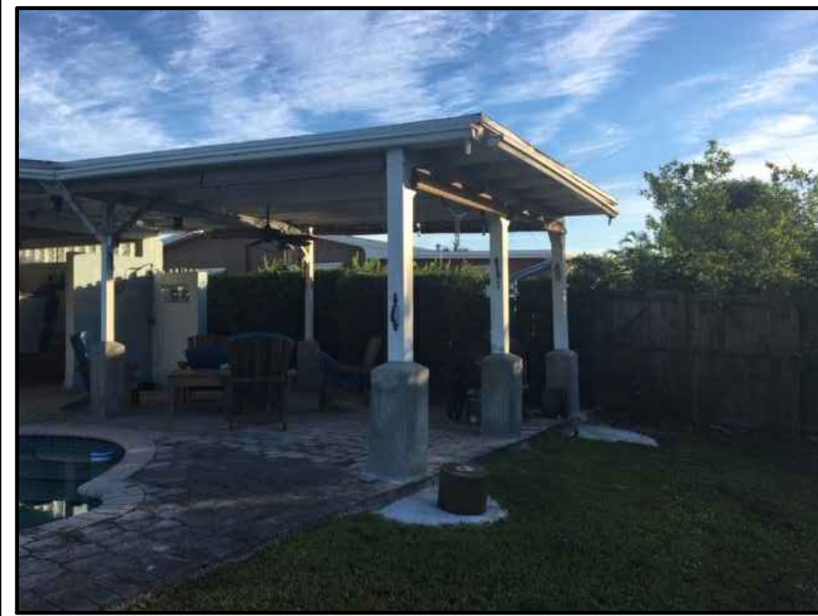
WEST TO PATIO ROOF
