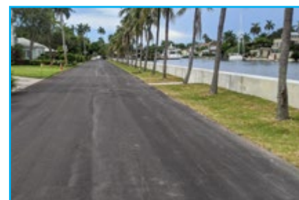
Newly elevated Isle of Palms Seawall
