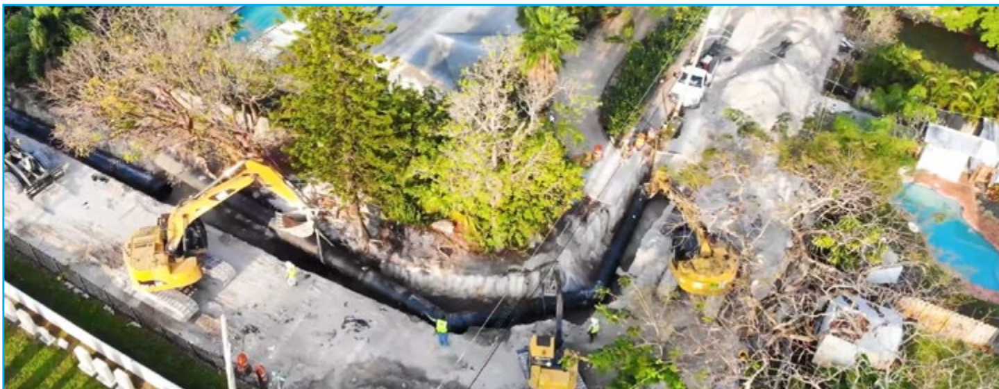
Installation of resilient infrastructure
