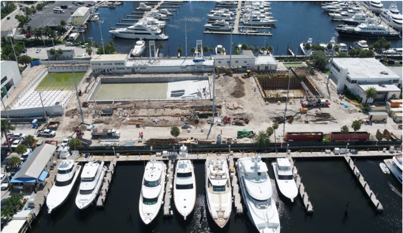
Aerial of Fort Lauderdale Aquatics Center Renovation Construction
