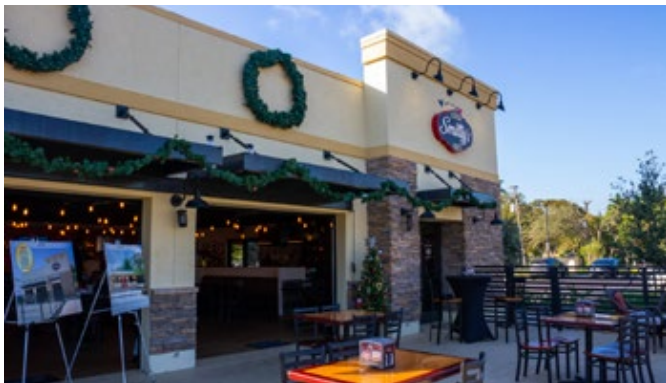
Completion of Smitty's Wings Restaurant
