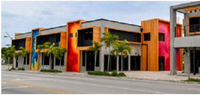
Completion of the Pharmacy Exterior
