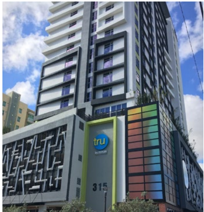
Completion of Flagler Village Hotel
