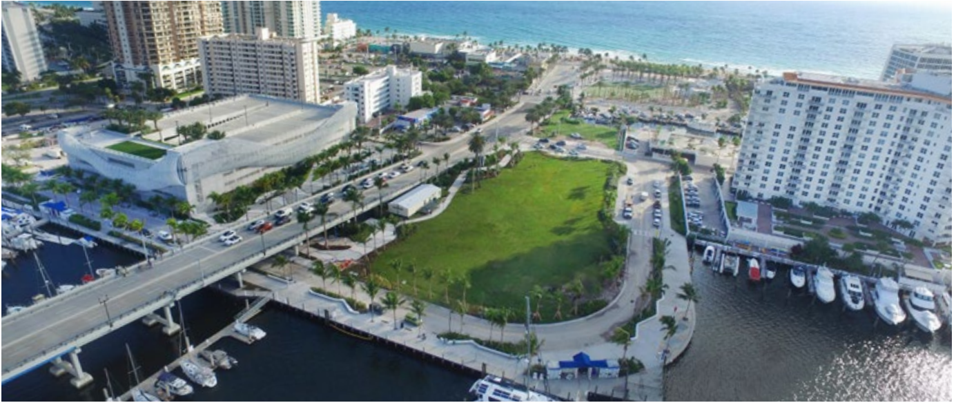
Aerial Las Olas Boulevard Corridor Improvement Project
