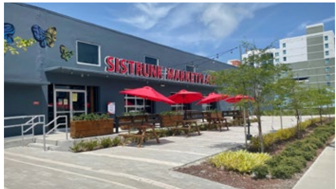
Completion of Sistrunk Marketplace Exterior
