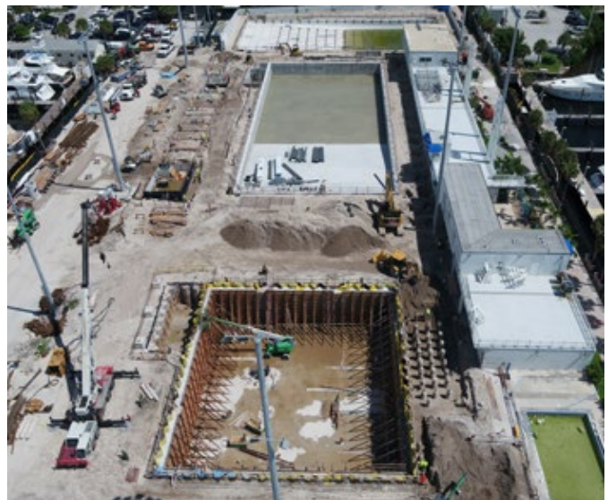
Construction of Fort Lauderdale Aquatics Center Renovation
