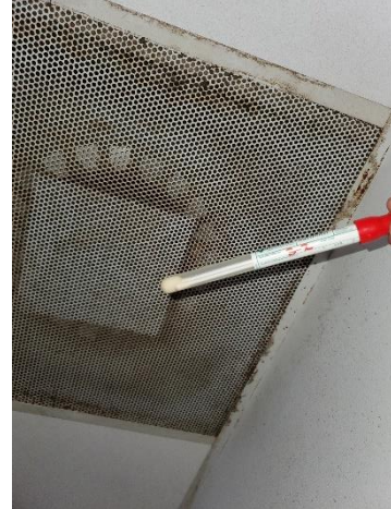
Photo 2: View of the A/C supply – Commissioners conference room.
