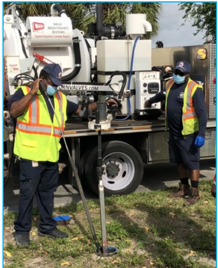
Photo of City crew inspecting and maintaining a water valve.
