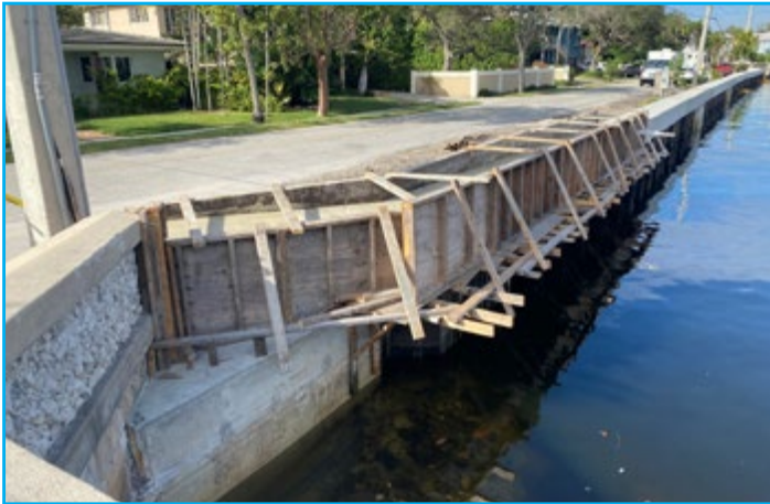
Cordova Road Seawall under construction
