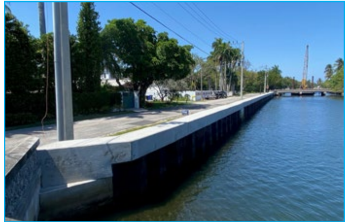
After photo of Cordova Road seawall
