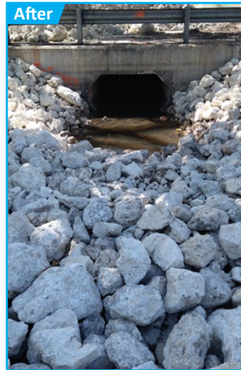
Melrose Park Drainage Culvert: Cleaned & Restored
