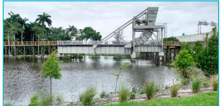
CSX Bridge and elevated walkway at River Oaks Preserve
