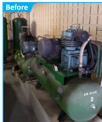
Before and after pictures of the Diesel Engine Air Start System
