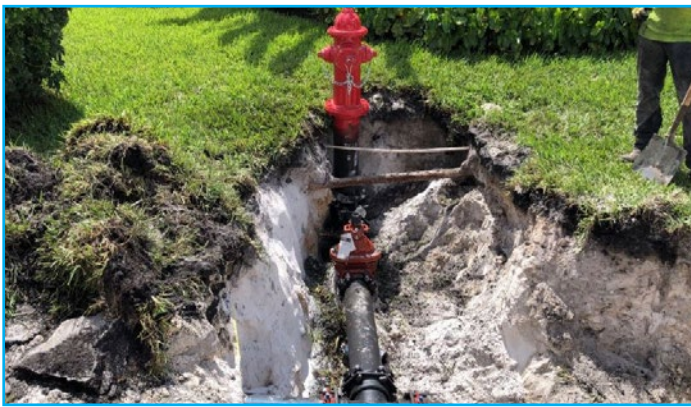
Photo Victoria Park Small Watermain Replacement
