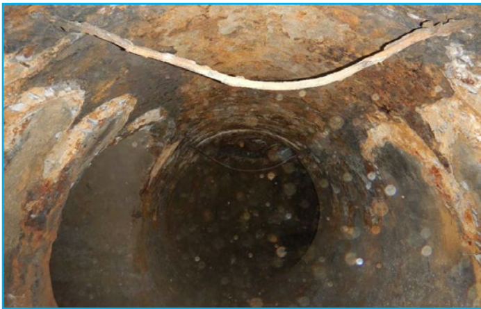
GTL PCCP pipe condition before CFRP Liner installation
