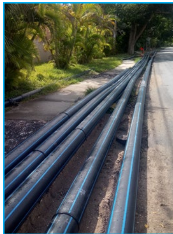
New HDPE Pipe Ready for Install
