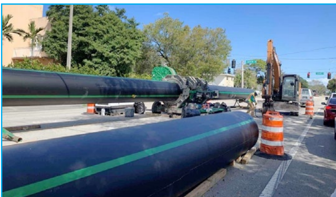
Installation of new Sewer Force Main on Northwest 13th Street
