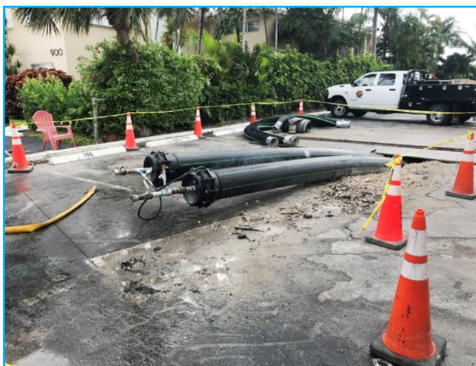
20-inch Diameter Pipe Sewer Force Main Replacement
