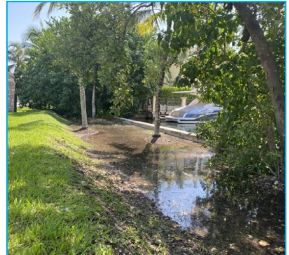
Figure 1 - King Tide overtopping seawall near San Marco and Las Olas Boulevard. With the milder king tides this fall, the earthen berm was adequate to prevent tidal impacts on Las Olas Boulevard. In preparation for future sea level rise, the City will be elevating this seawall in the next 18 months.
