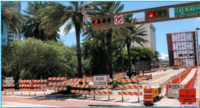
Sample MOT plan in effect for Andrews Avenue Drawbridge rehabilitation.
