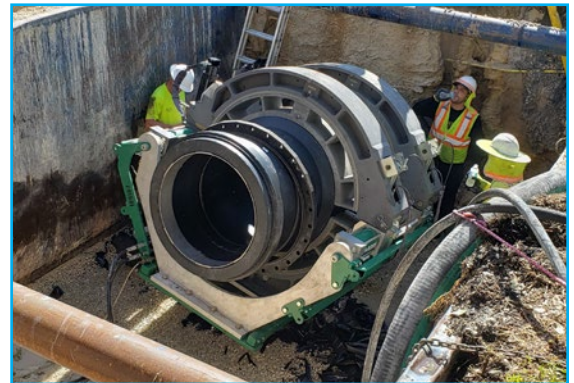
Fusing Pipe Connection
