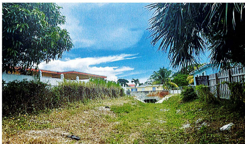
Figure 5: Grass and Weeds Growing between the Chain Link Fence Facing the Ditch and a Second Fence Facing the Private Property.
