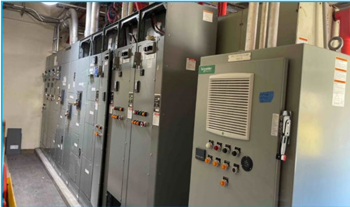
Installation of New Motor Control Centers
