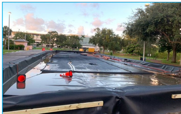
Photo showing area where crews pumped the dredged sediment for processing
