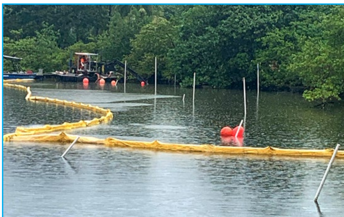
Photo of dredging during the George English Lake Restoration Project
