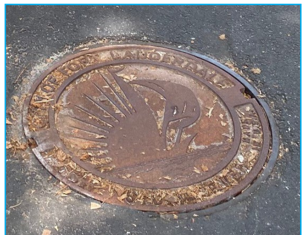
Fort Lauderdale Manhole Cover
