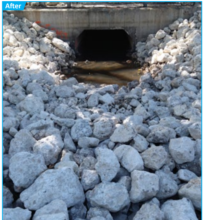
Melrose Park Drainage Culvert: Cleaned & Restored
