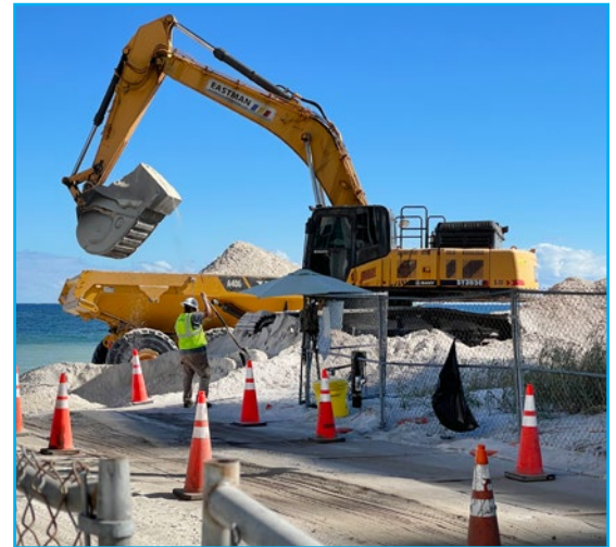
Crews are currently adding sand to Fort Lauderdale Beach
