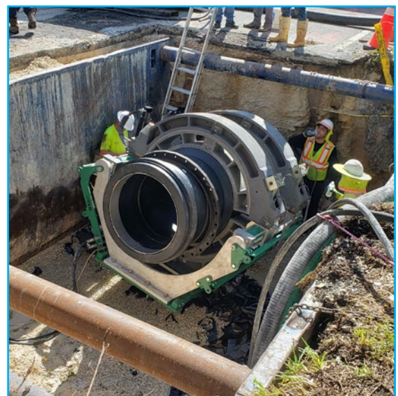
Fusing Pipe Connection
