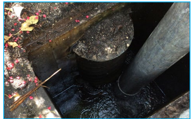
Cleaning a catch basin containing a pollution control baffle
