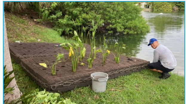
Floating Treatment Wetland in Lake Melva
