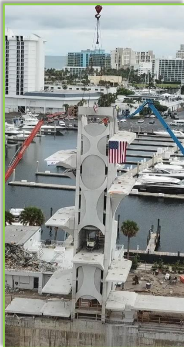
The dive tower under construction
