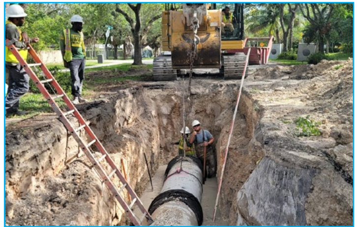
Ongoing stormwater improvements in Edgewood
