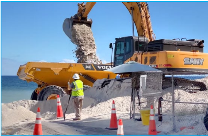
Beach renourishment on Fort Lauderdale Beach
