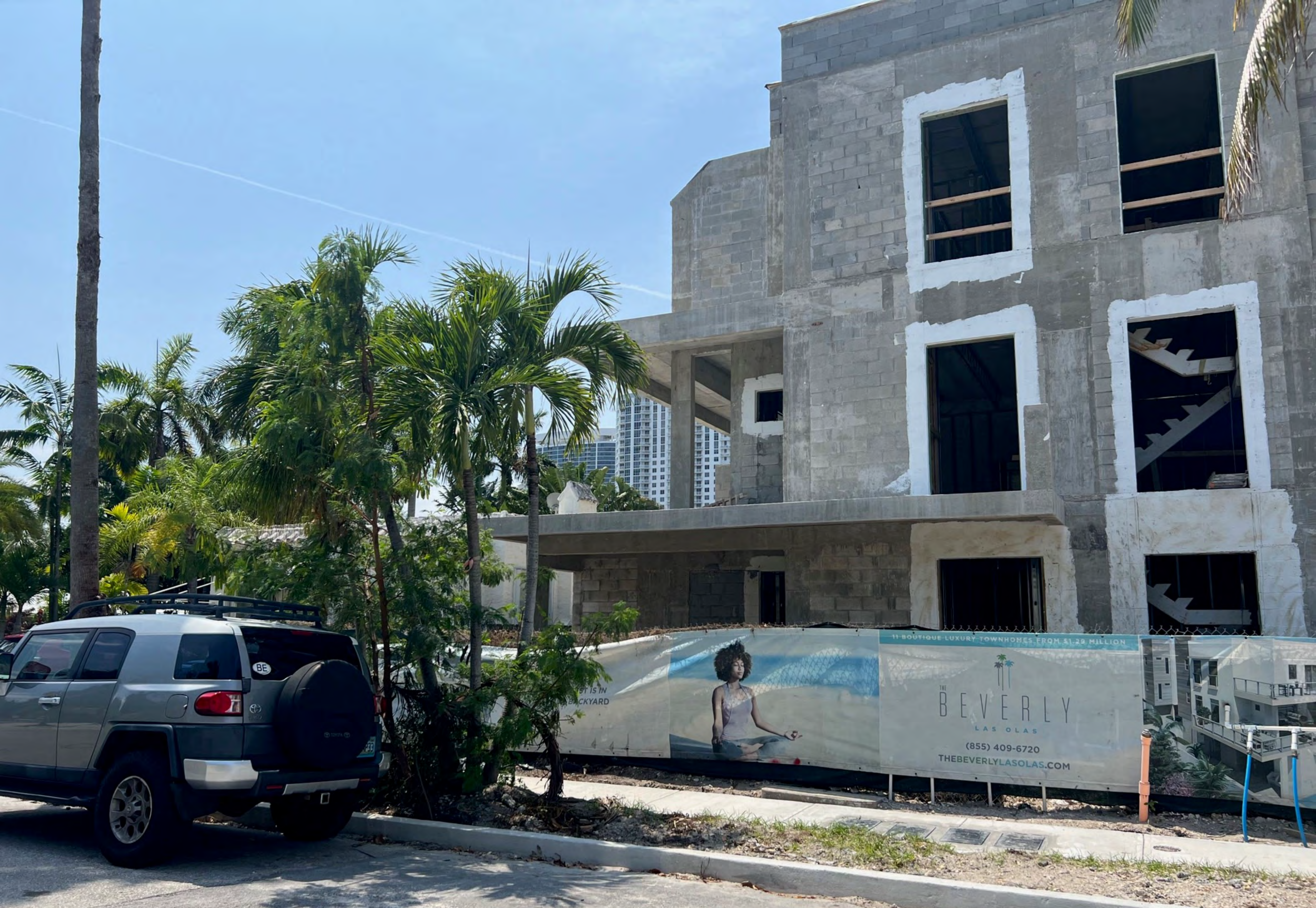
View Looking West SE 11th Avenue
