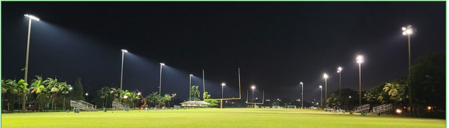
Photo of a Mills Pond Park field that shows new LED lighting on the left side and halide lighting on the right side
