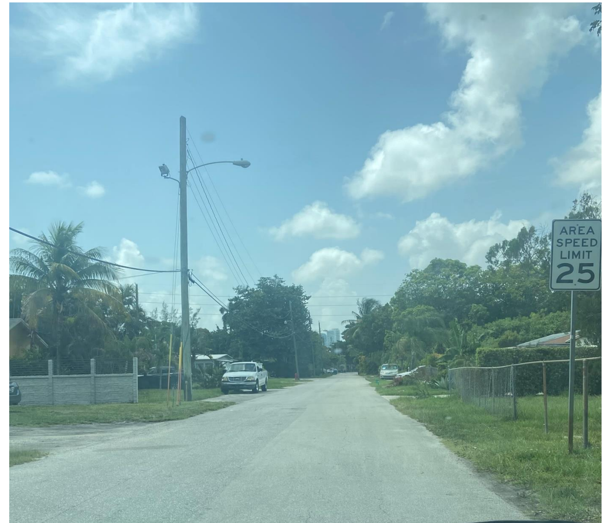
View to the South
