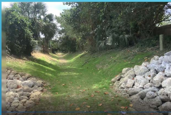
Grass seed applied in the drainage ditch
